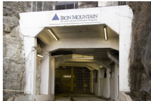
Entrance to Iron Mountain underground facility.
